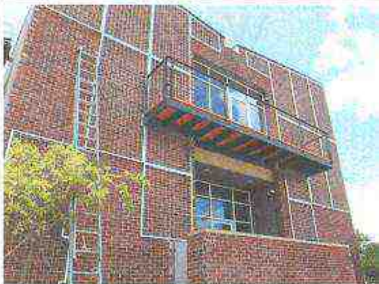
At top, recycled wood from its own building was used to make a conference table for PeopleMatter in Charleston. Charred wood makes a unique inlay. Bottom, reclaimed brick is used on the facade of the building for Biz611 in Hendersonville, N.C. Photos/Jorge Riano, GreenBy3
