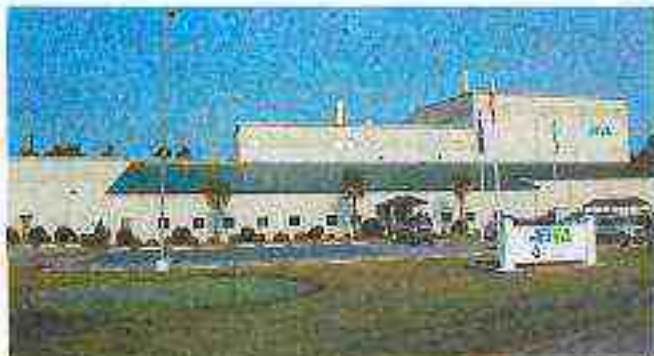
VIVA Recycling Facility in Moncks Corner, SC
